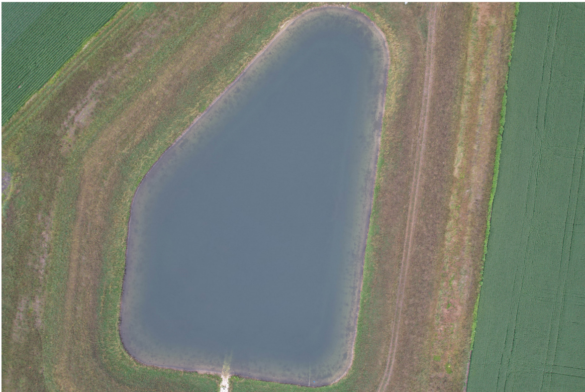
Aerial view of the drainage water recycling reservoir at the Dayton site filled from pumping water from an adjacent county drainage main.
